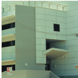
M.R.D Tunnel Control Building
